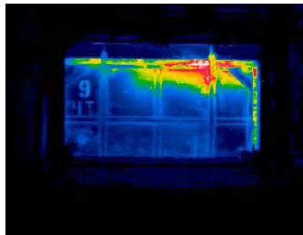
Furnace Door Seal
